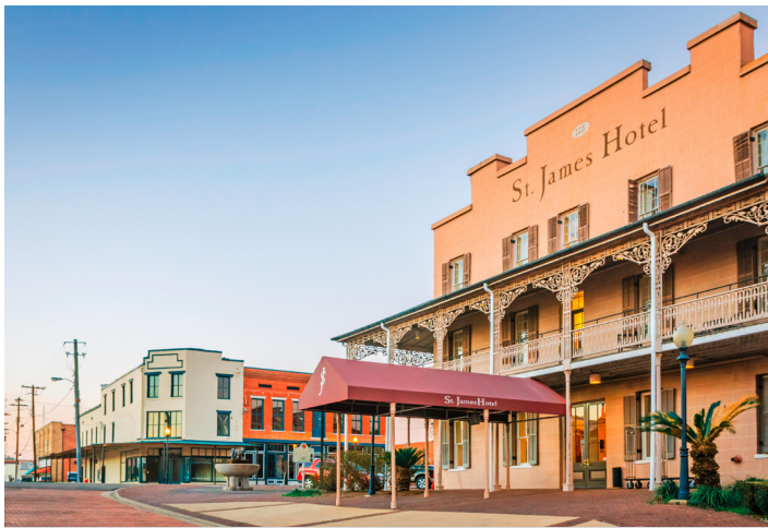
American South Fund Management funded renovations of the St. James historic hotel in Selma, Alabama, now part of the Hilton-branded Tapestry Collection. (Betty Johnson)
